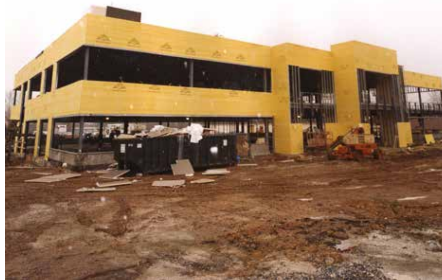
Construction of the new building, 2290 Butler Pike, Plymouth Meeting, Pennsylvania
